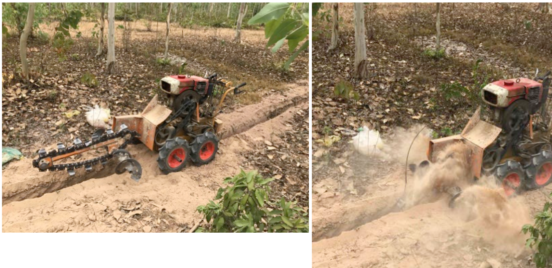
Above and below: mechanical trench digger installing a water pipe network.
