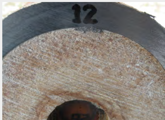
There was no evidence of water ingress at this cut point, and no corrosion visible on the inside of the casing
