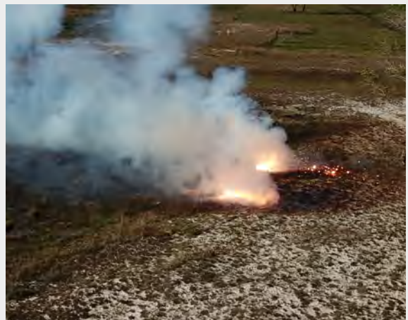
Burning out the main bodies of the 2 x Mk 82 500 lb bombs; the burnout lasted 22 minutes
