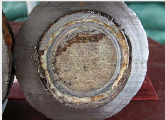
Water entering the casing through the fuze well has caused corrosion of the inner assemblies, causing a build-up of expanded rust and aluminium oxide
