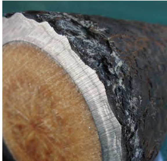
The corrosion of thick steel casings is normally superficial, but may make it hard to measure the calibre
